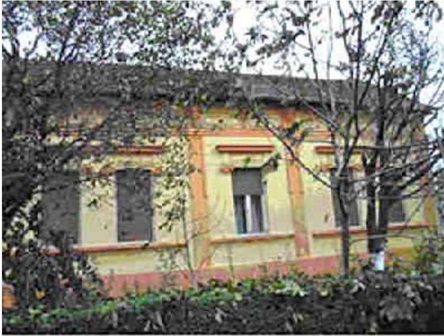
Picture 12 – A modernised half-transverse house in the Water Lane.
